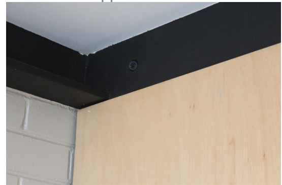
Pinhole camera with separated camera body for discrete application in a showroom
